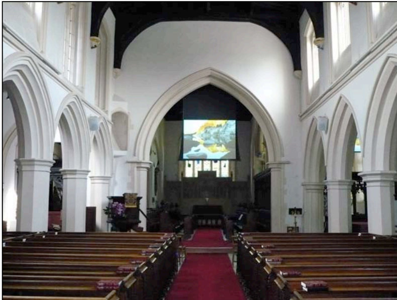
A custom designed long-drop tab-tensioned screen was commissioned for St Mary's to provide clear visual communication and the ultimate in discreet installation. Actual image – not superimposed.
