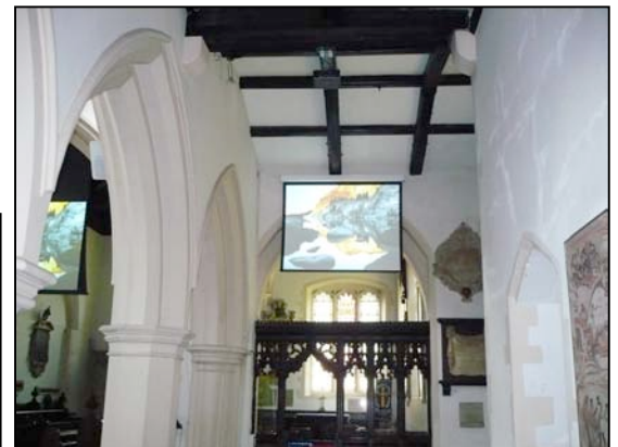
One of the two side aisle screens featuring 3000 lumen Eiki projectors and remotely operated motorised screens
