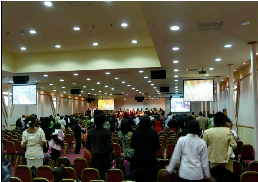
An RCCG Victory House service in progress showing ceiling mounted EV RX series speakers, Eiki digital projectors and motorised screens
